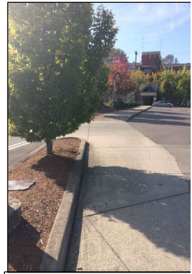
The pedestrian path is a different color and texture, however its ends do not line up with the actual path pedestrians were observed taking.
