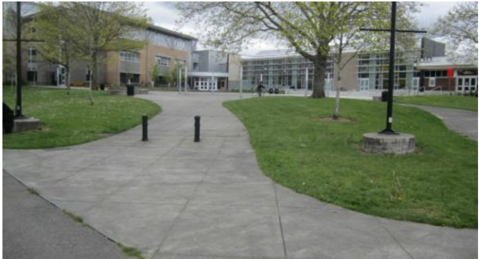
The Community Center and South Shore K-8 Campus is open, inviting, and easy to see into and out of during the day.
