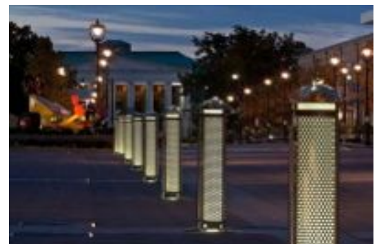
An example of excellent lighting in a public plaza in South Carolina. It helps define the space, and casts even, reflected light along the pathways.
